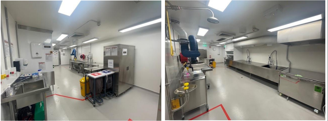
The refurbished laboratory (Photos by Ronda Eastall)
